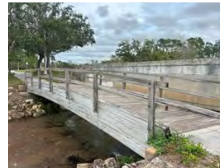
Shared-use path along Sumter Blvd
