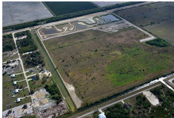
Aero Photo 727.520.8181 www.aerophoto.com Caloosahatchee River Estuary Storage & Treatment - CREST Dh II Image # 42 Date 02.13.24
