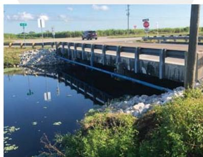
The bridge carrying Airglades Boulevard over Cessna Canal in Hendry County had significant channel contraction scour, causing undermining to the abutments and approach slabs. For this project KCA staff performed a field
