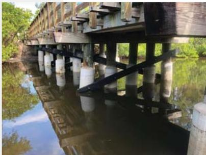
The Legacy Trail Pedestrian Bridge over Hatchett Creek (Bridge No. 4535), located in Sarasota County, was exhibiting areas of severe deterioration to the substructure. This pedestrian trail bridge exhibited severe marine borer damage to the
