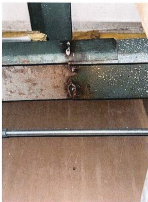
Pulin's Welded Connection Corrosion (PEMB)
