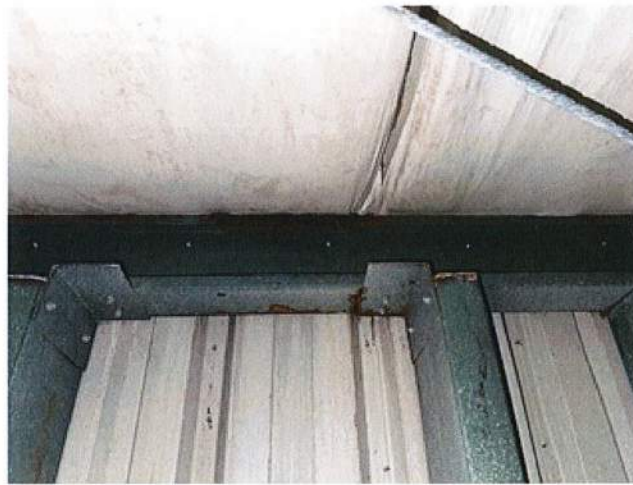
Perimeter Purlin Corrosion (PEMB)
