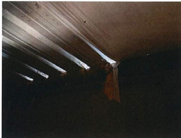
Exterior Roof Panel Openings / Interior Exposed to Elements / Purling Corrosion
