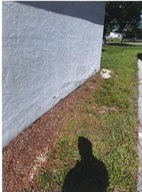
Bulging in Stucco Finish (Masonry Structure)
