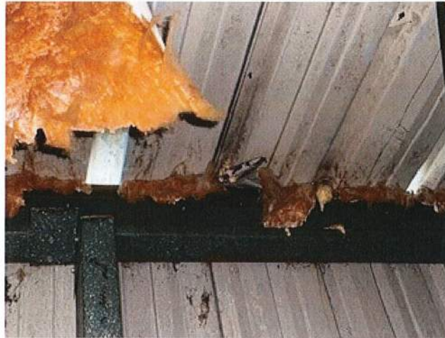
Perimeter Purlin Corrosion / Openings in Roof Deck / Interior Exposed to Elements (PEMB)
