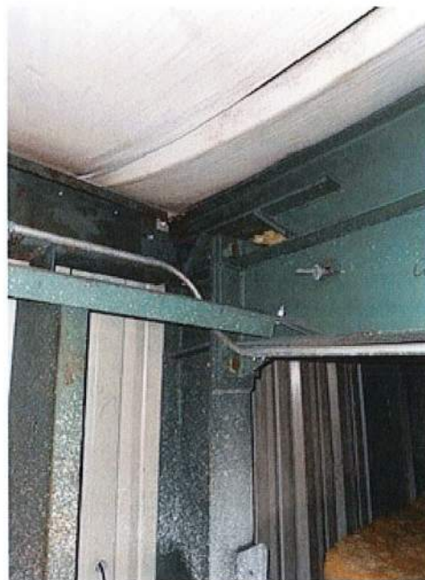
Purlin to Building Frame Connection Corrosion (PEMB)
