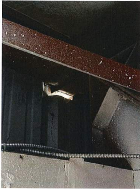
Exterior Wall Panel Opening / Exposing Interior of Bldg. to the Elements (PEMB)
