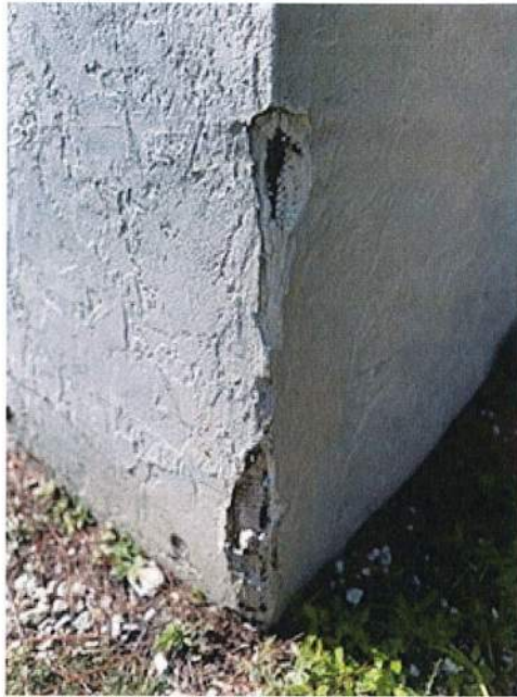
Stucco Finish Chipped Away at Corners (Masonry Structure)
