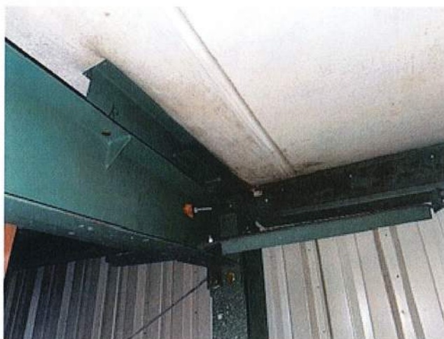
Purling to Building Frame Corrosion Connection (PEMB)
