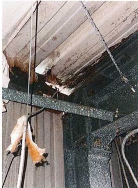
Exterior Wall Panel Opening / Exposing Interior to Elements / Corrosion at Purlin and Bldg. Frame (PEMB)
