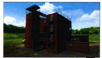
Public Safety Training Complex
