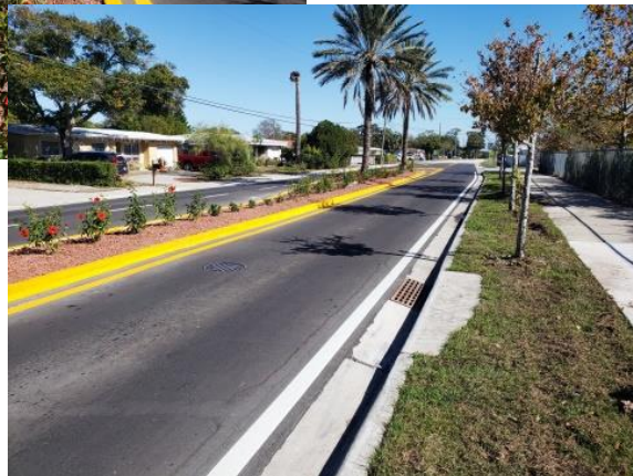
Median Lane Modifications Landscaping and Irrigation
