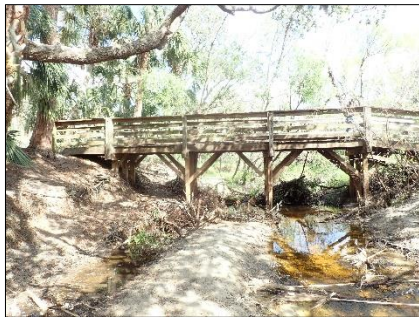
MCEP Equestrian Bridge Replacement
