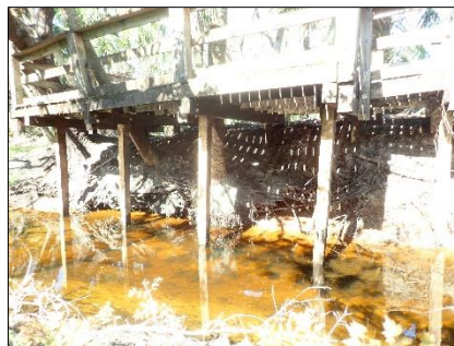
MCEP Observation Deck Repair
