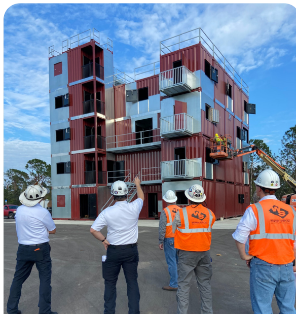
In Progress: City of North Port - Fire Training Tower
