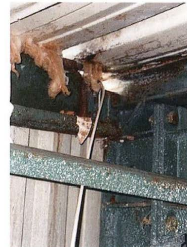
Exterior Roof Panel Openings / Interior Exposed to Elements / Corrosion at Purlin and Bldg. Frame (PEMB)
