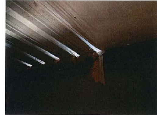
Exterior Roof Panel Openings / Interior Exposed to Elements / Purling Corrosion
