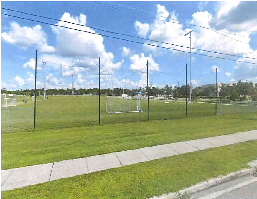
Pre-storm Photo of Northern Street Netting GPS: 27.070487, -82.224148
