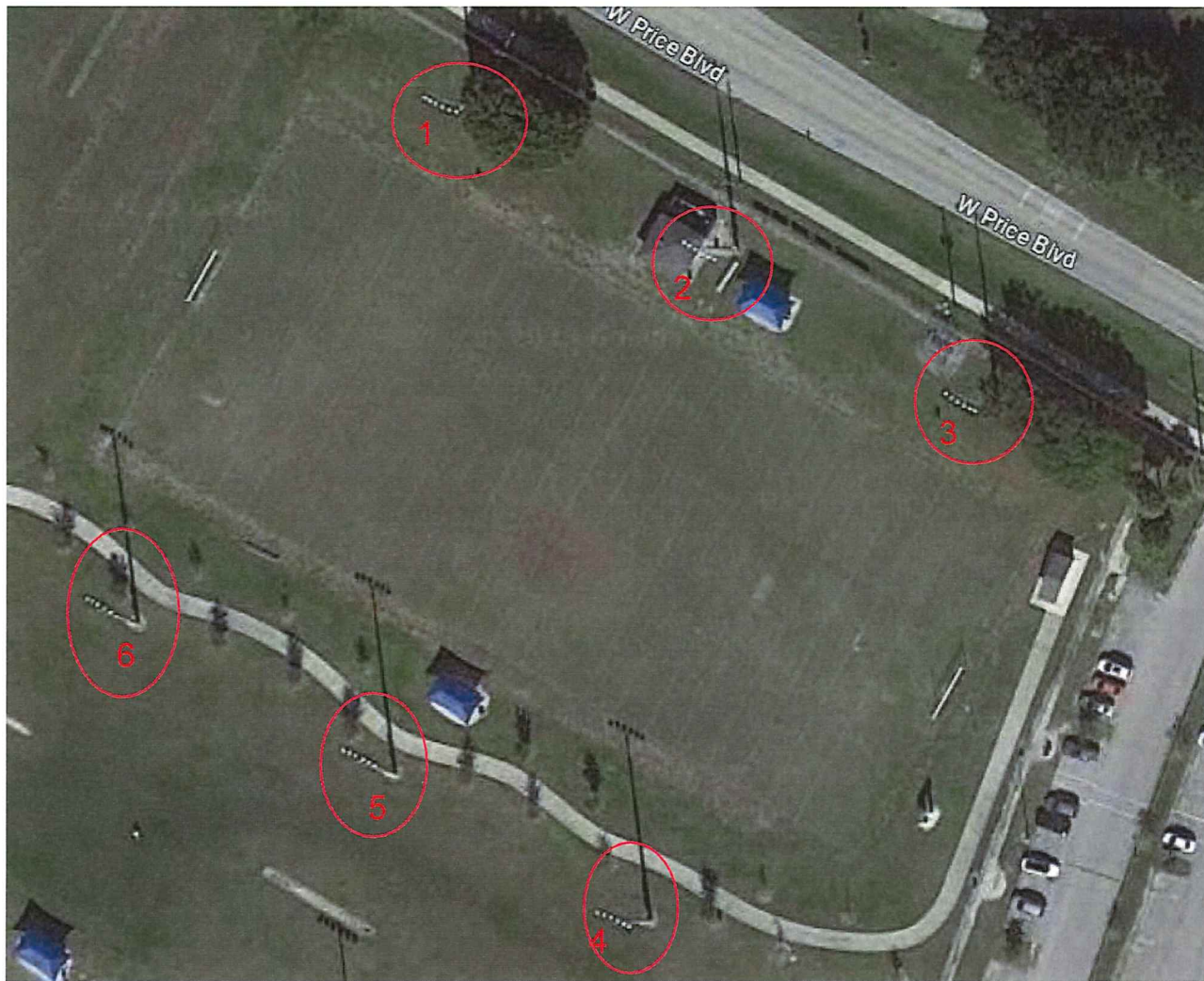
Field 4 Lighting Aerial
