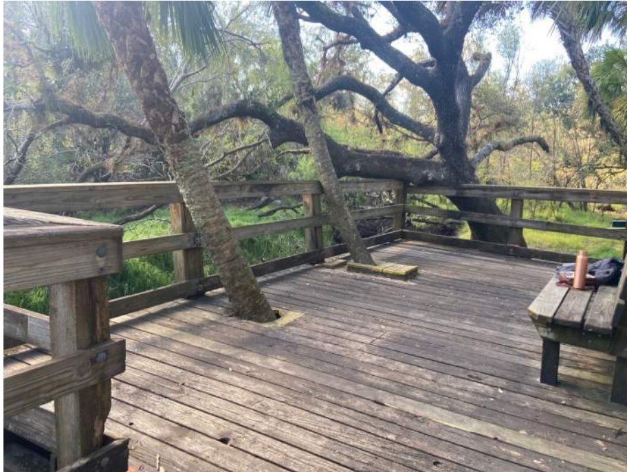
Photograph #11: Overall Observation Deck
