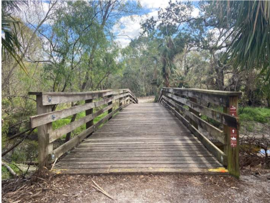
Photograph #1: Overall Equestrian Bridge
