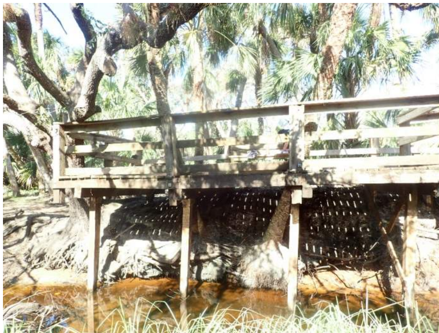
Photograph #12: Piles on Water
