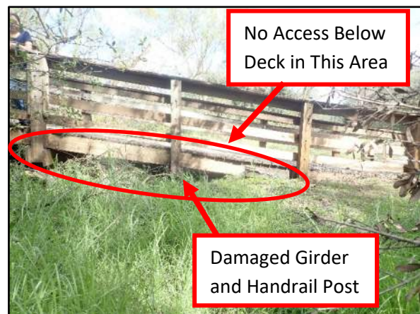
Picture 2 – Southeast Entrance Of Bridge
