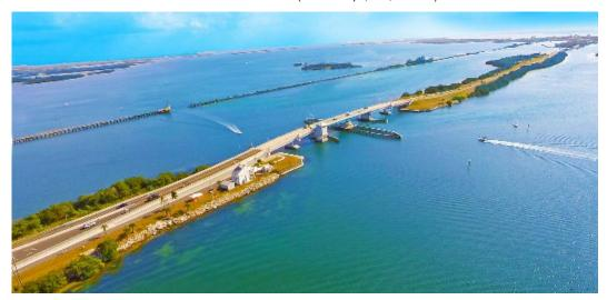
H&H provided comprehensive design services for replacement of the Gasparilla Island Swing Bridge, including field inspection, a PD&E study, complete design, and post-design engineering support. The PD&E study provided details on high-level fixed, swing, and bascule alternatives on north and south parallel alignments. A swing bridge on a southerly alignment was chosen to minimize environmental impacts to seagrass and mangroves and as to satisfy the SHPO Memorandum of Agreement.
