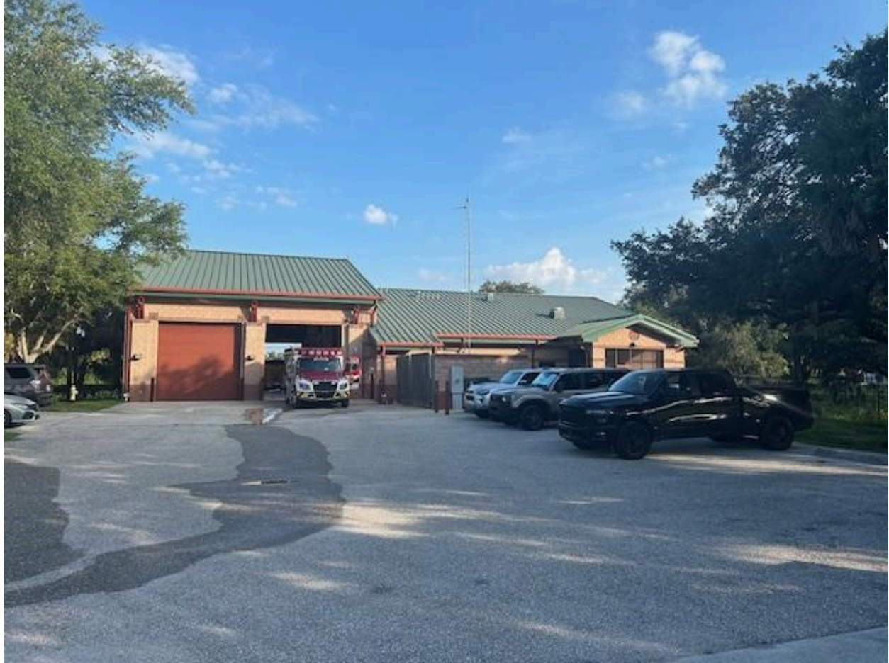
Fire Station 83 Rear
