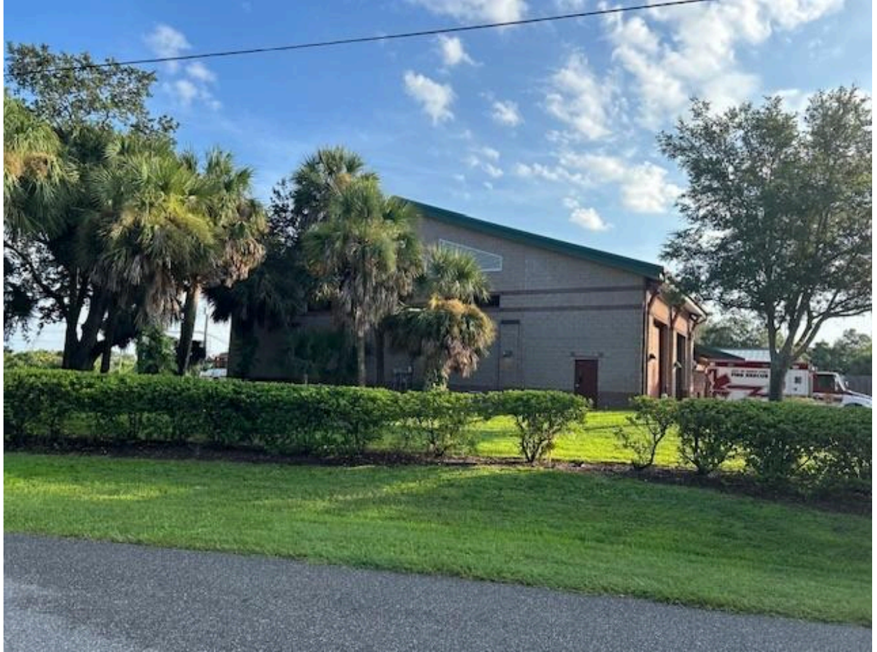
Fire Station 83 Side from SW
