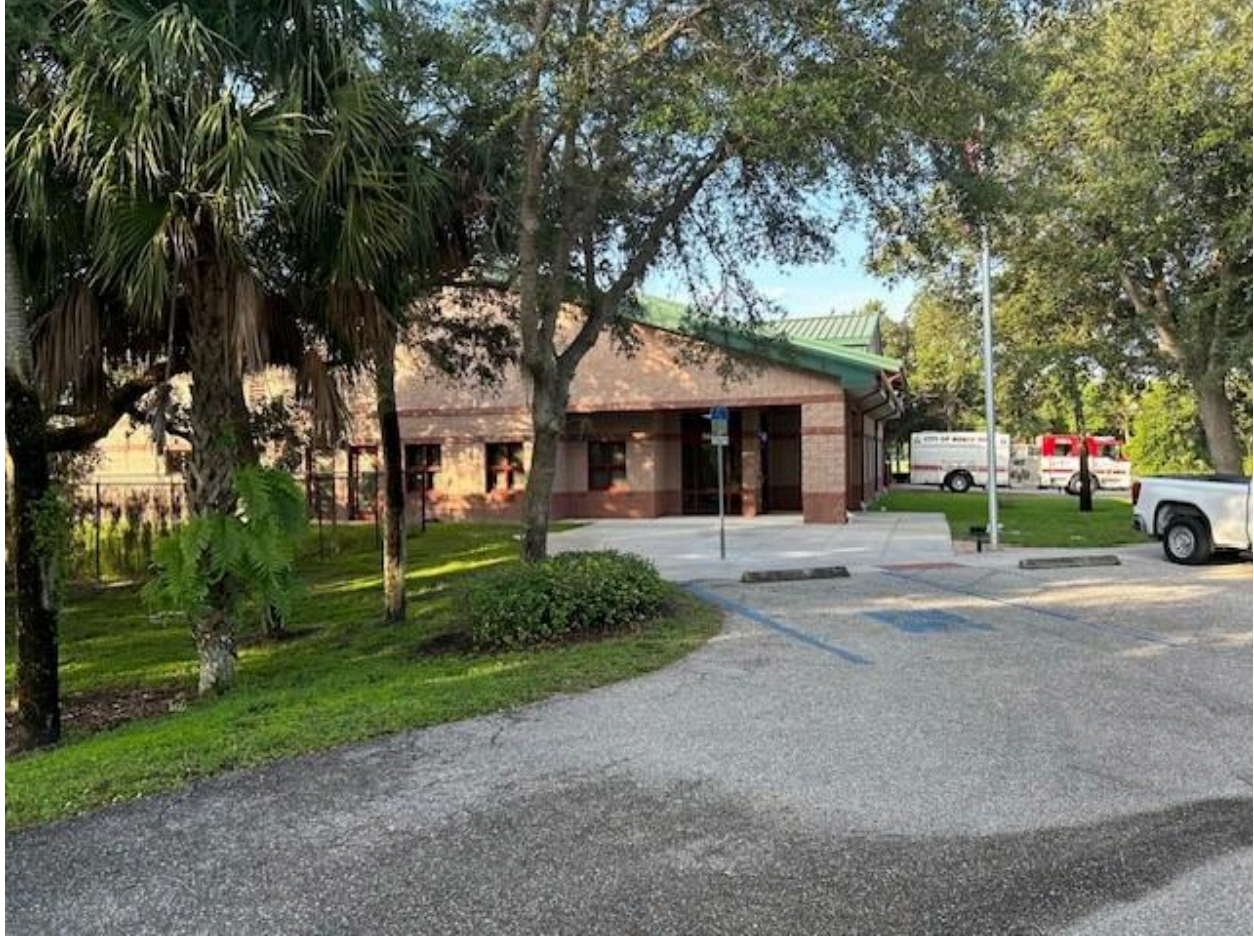
Fire Station 83 Side from North East
