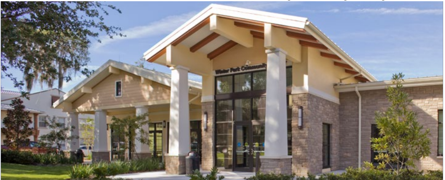
Community Center Designed for a Florida Municipality City of Winter Park Community Center
