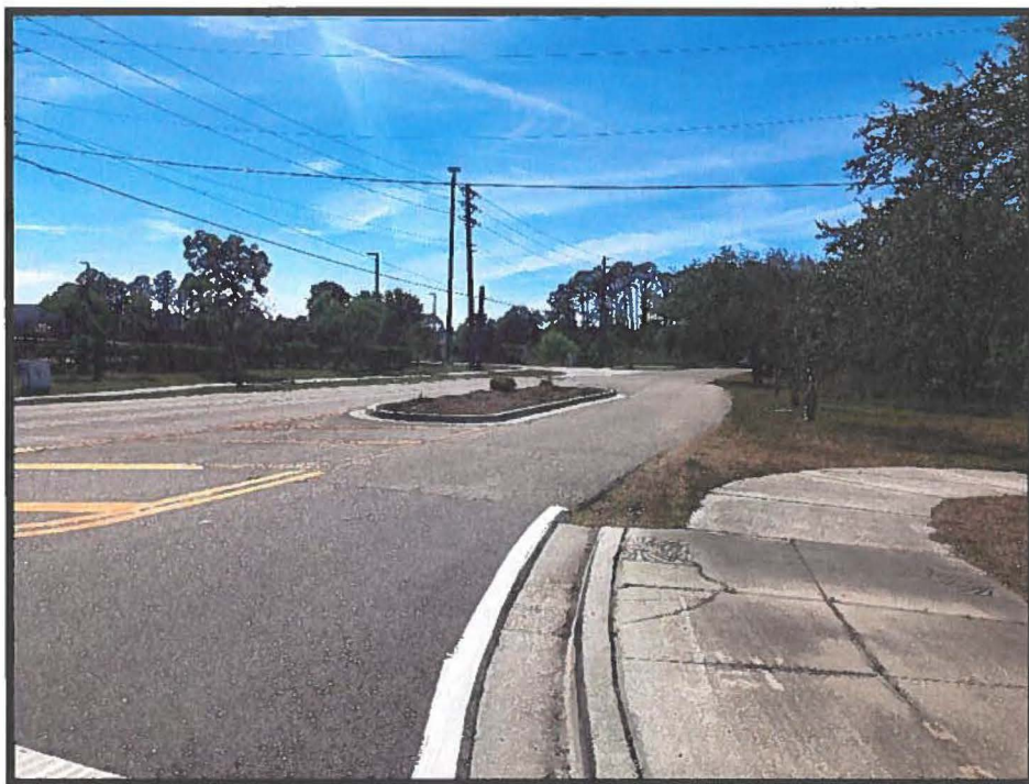
Commerce Parkway, looking west
