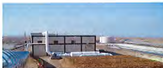
Synagro utilizes an enclosed biosolids receiving and mixing building along with biofiltration in its compost system that controls VOCs and odors for the surrounding area.
