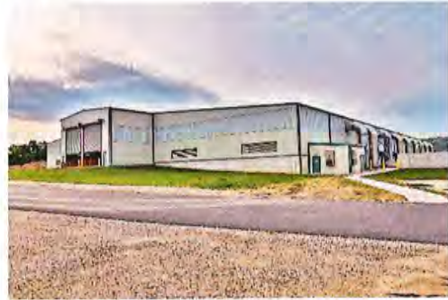
The Cumberland County Organics Recycling Facility was designed to utilize renewable energy, creating a highly sustainable, environmentally and community-friendly solution.
