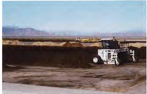
With operations encompassing 40 acres, AS Soils is one of the largest outdoor biosolids composting facilities in the U.S.
