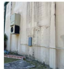
FIGURE 13. WATER DAMAGE AT EAST FACADE
