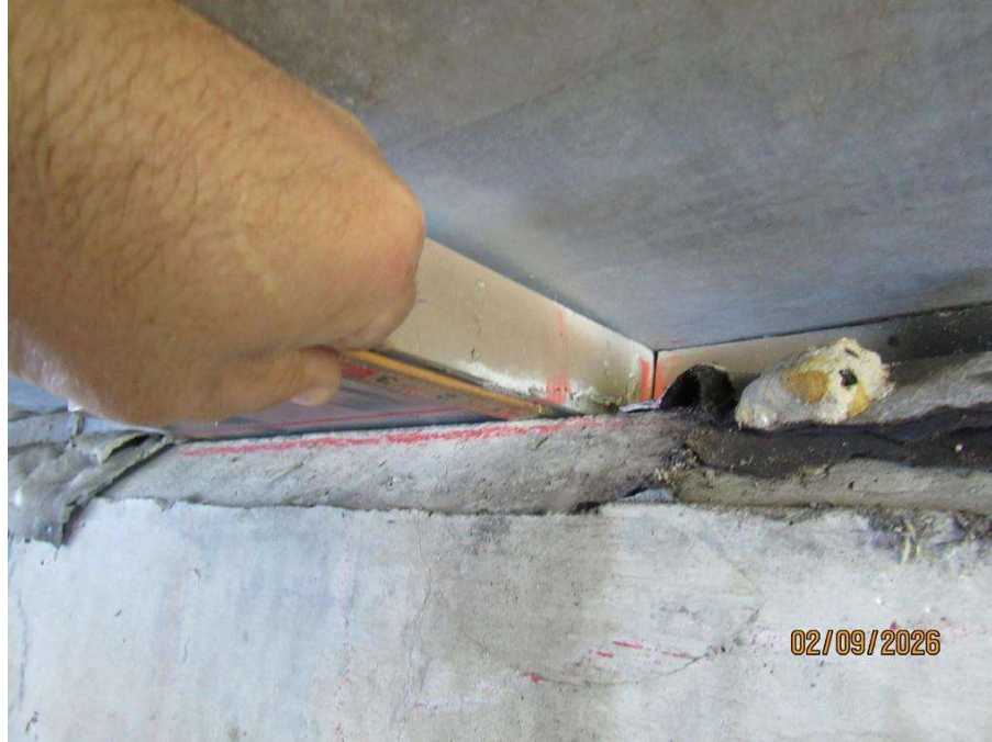
Photo 4: Bearing 1-9 walking out.
