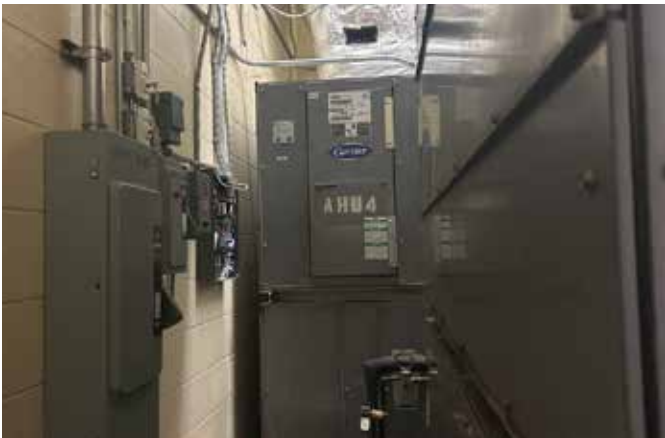
Air Handling Unit and Power Supply
