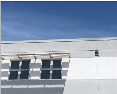
Gulf Gate Elementary School Improvements
