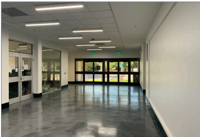
USFSP Harbor Hall Renovation
