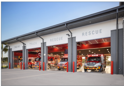
North Port Fire Station No. 86
