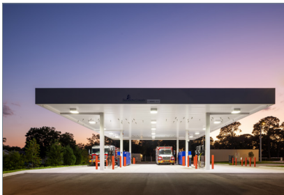
SRQ Fire Station No. 9 Fueling Facility
