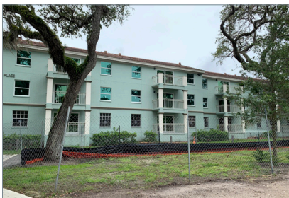
RCAD - Whitaker Bayou Studios Renovation
