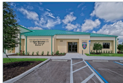
East Manatee Fire Rescue Station 7
