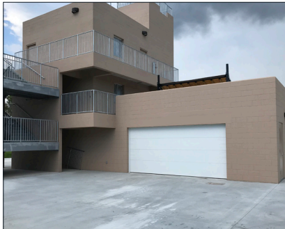
Cedar Hammock Fire Training Tower
