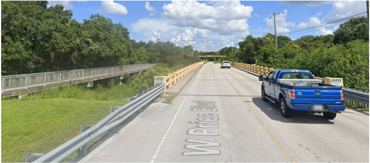
Existing Roadway and Pedestrian Bridge Viewed from West End, Looking East
