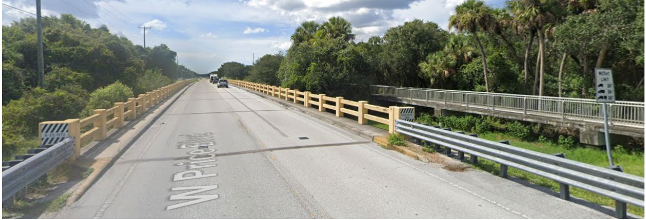
Existing Roadway and Pedestrian Bridge Viewed from East End, Looking West
