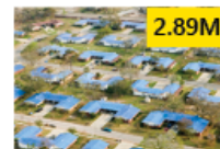
Gulfport, MS Hurricane Katrina, '05
