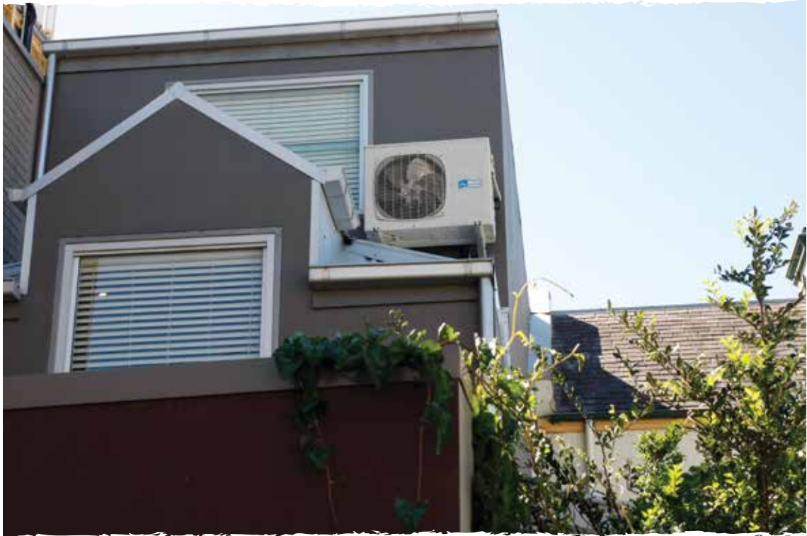
Air conditioner outdoor unit placed so as not to annoy neighbours. Photo: EPA
