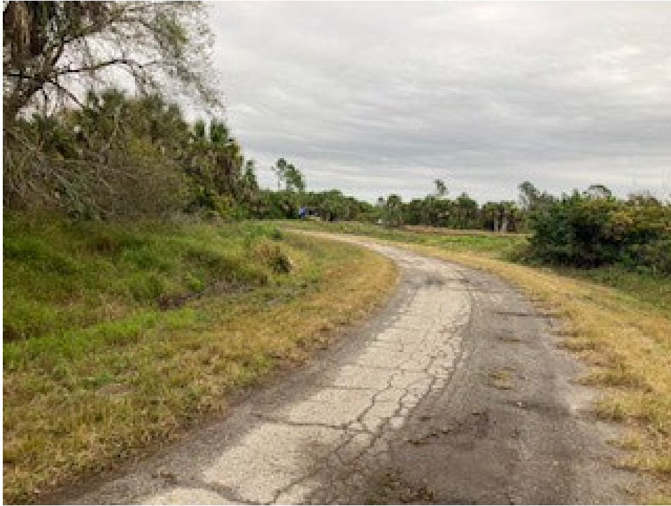
Silverleaf Road, Looking east
