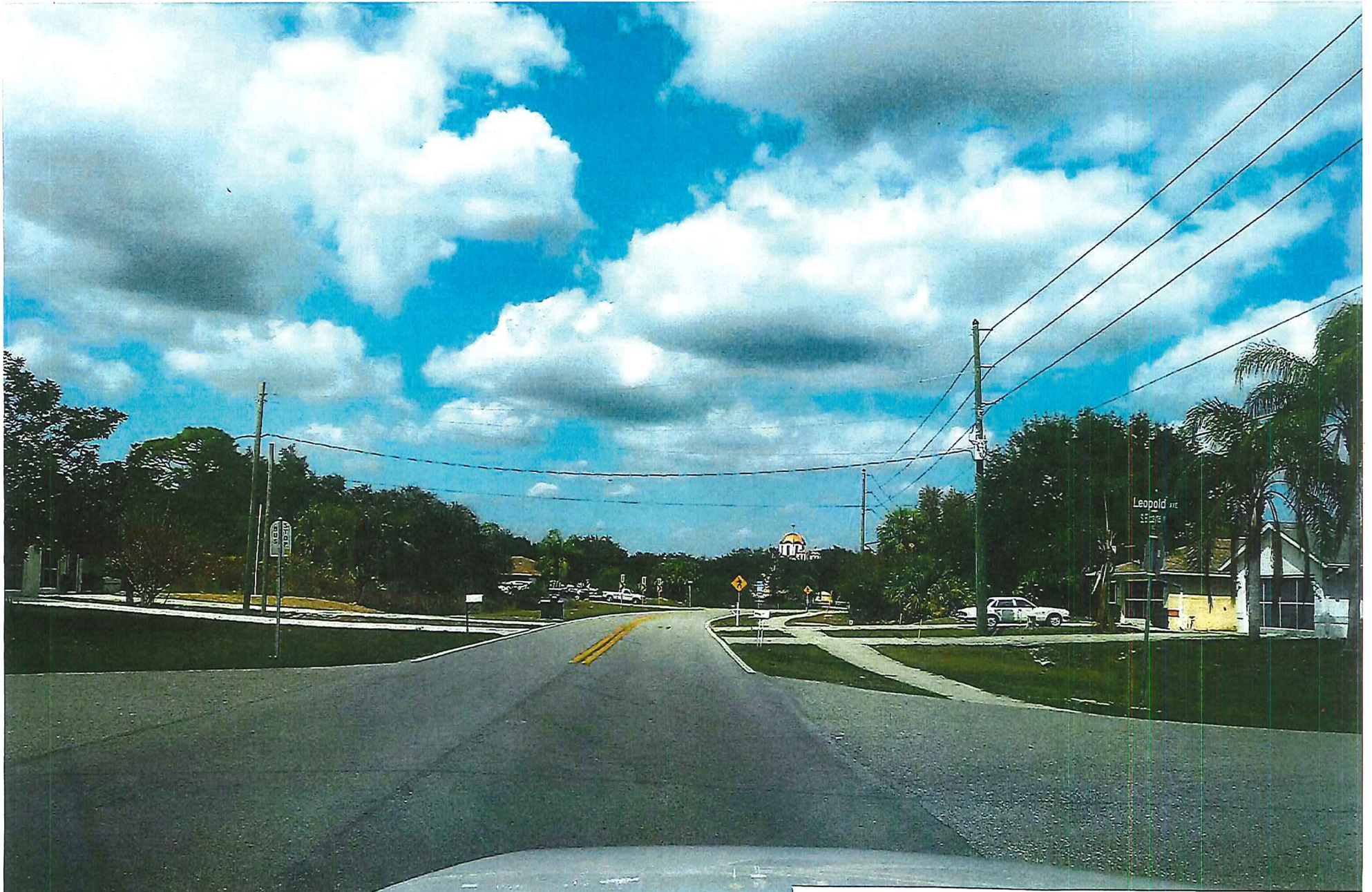
EXHIBIT #7 BISCAYNE DRIVE – EXISTING CONDITIONS Looking north from Leopold Avenue (02/02/17)
