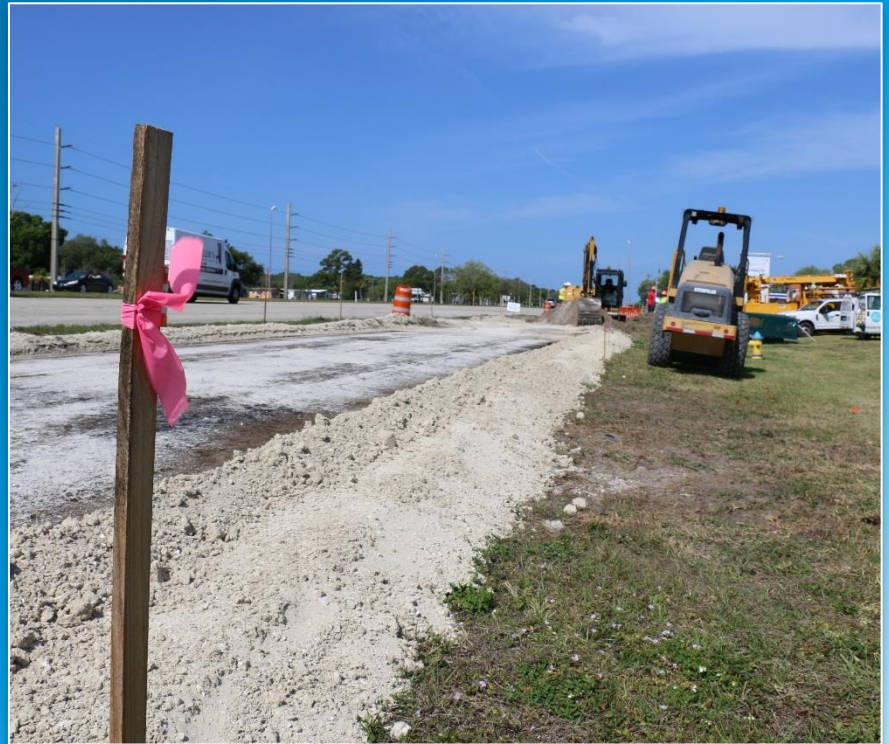
Infrastructure construction, previous project on US 41
