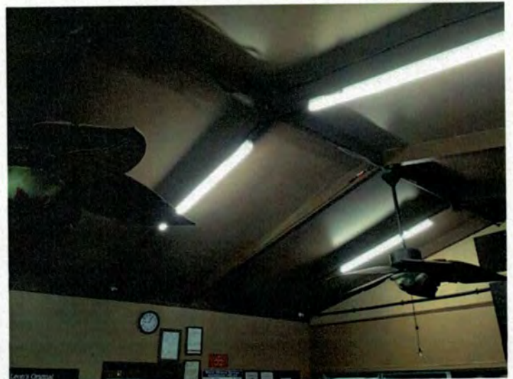
Interior of spa building
