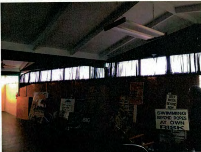
Interior of meeting room showing folded plate roof configuration with non-bearing walls and clerestory glass
