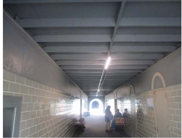
Picture 14 Building 2 - Breezeway Looking South. Ceiling Joists.
