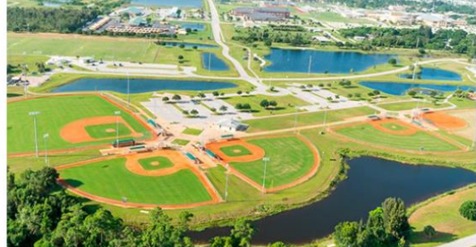
FIGURE 5.3A The Village Park may include a variety of sports fields, playground and passive recreation connected by walkways and bike trails. Photo example shown.
