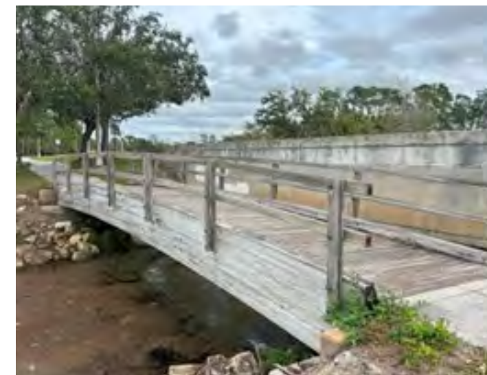
Shared-use path along Sumter Blvd
