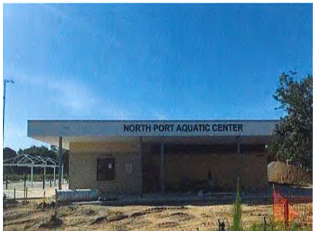
Facility signage is being completed.
