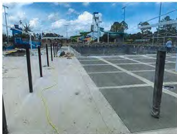
Concrete is being poured for the pool deck.
