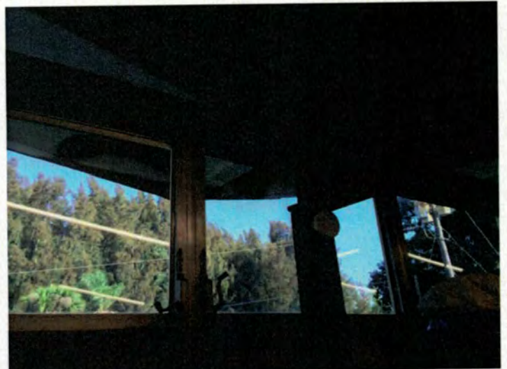
View of steel post and beam construction
