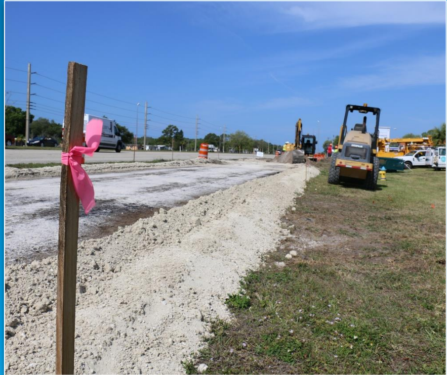
Infrastructure construction, previous project on US 41
