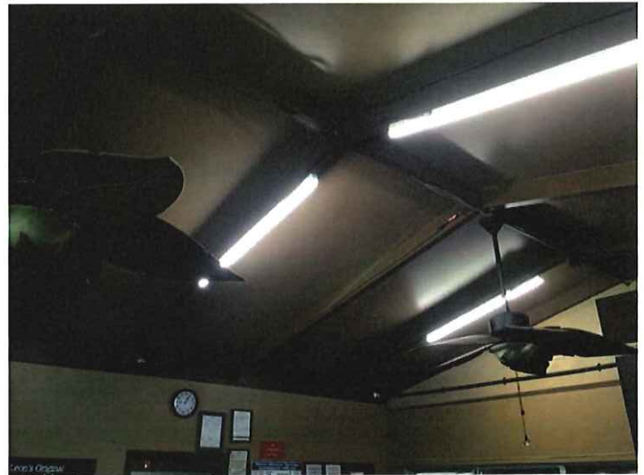
Interior of spa building
