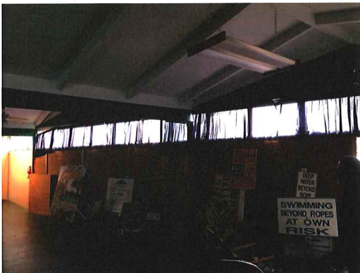
Interior of meeting room showing folded plate roof configuration with non-bearing walls and clerestory glass
