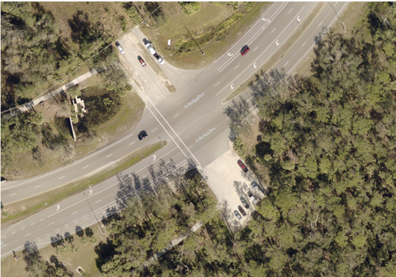
The southern parcels of the Core Activity Center are connected to Sumter Boulevard with driveway stubs. Source: Sarasota County aerial imagery
