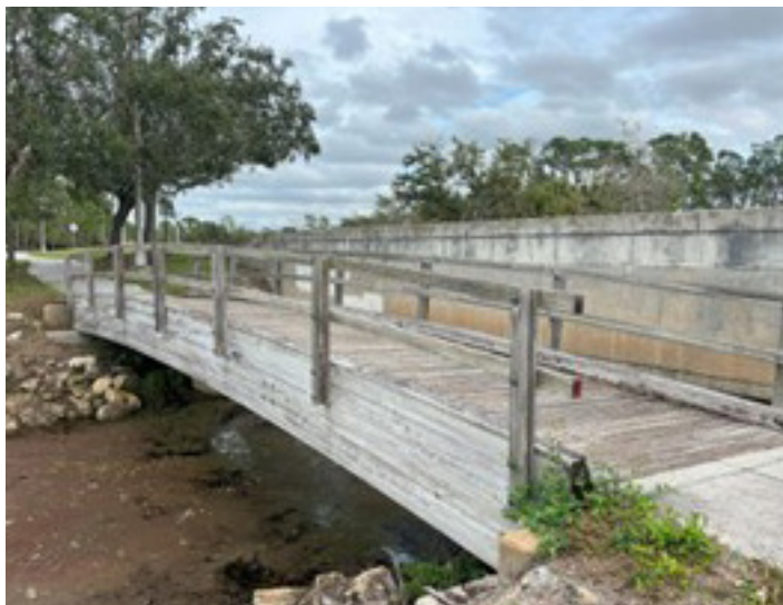
Shared-use path along Sumter Blvd
