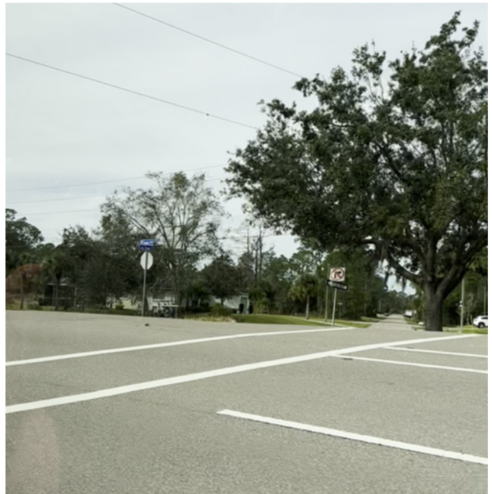
Existing intersection of Sumter Blvd. and Lady Slipper Ave.
