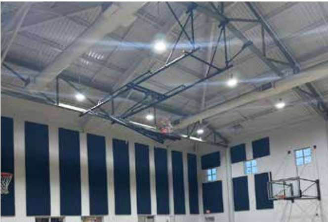
Gymnasium Exposed Structural and HVAC System
