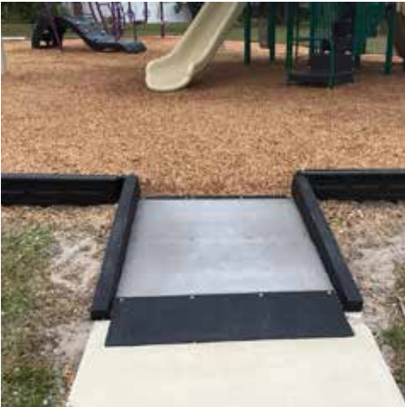
ADA Accessible Entrance
