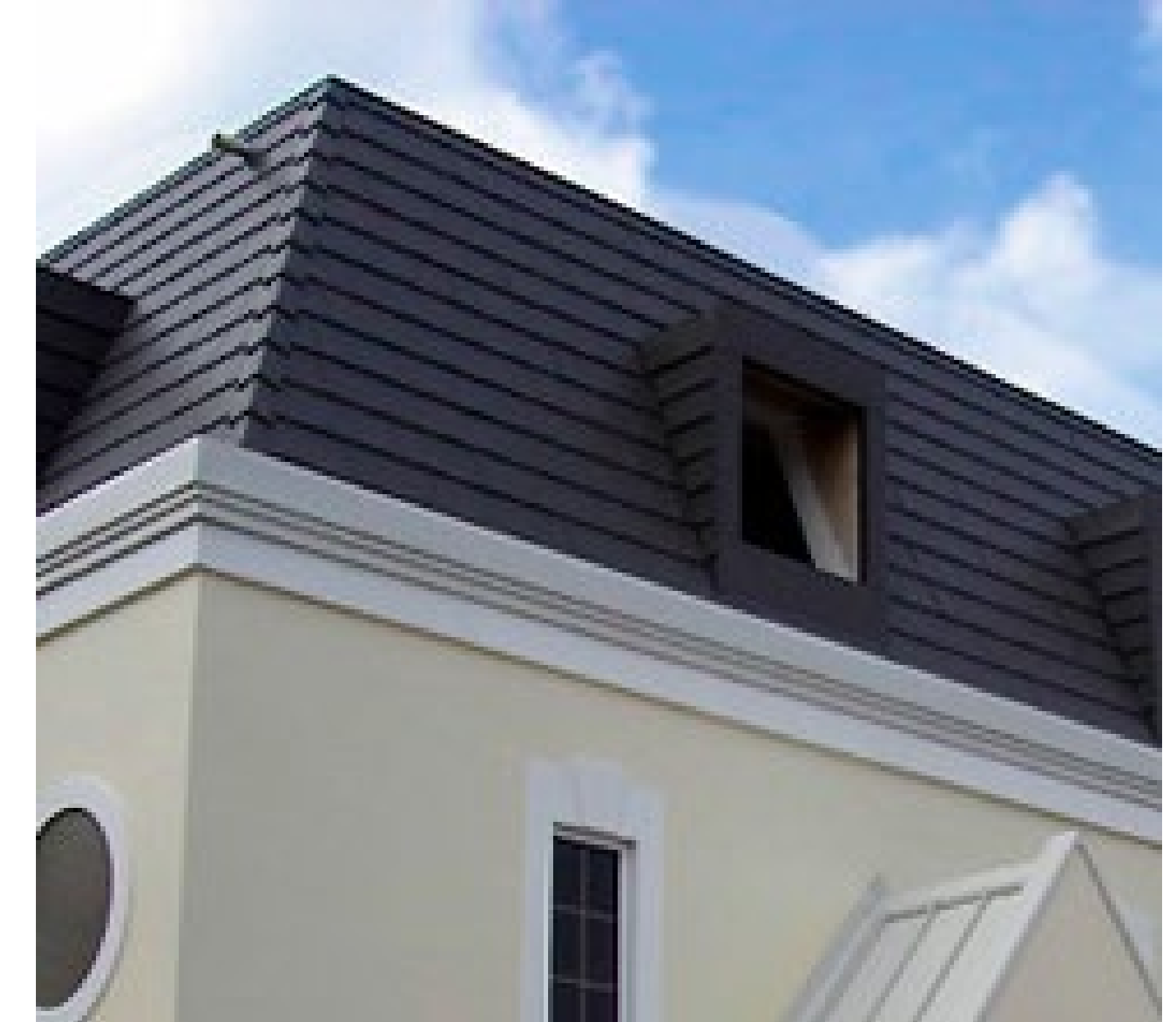
FIGURE 11.5.1.B Non-residential and multi-family buildings may have flat roofs but should use a mansard wall to screen edges and mechanical units.
