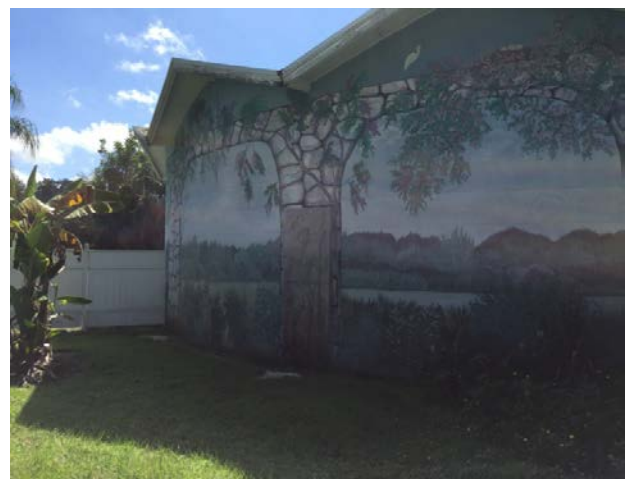
Picture 18 Building 3 - Cyclorama Stucco
