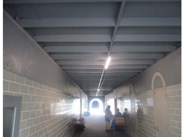
Picture 14 Building 2 - Breezeway Looking South. Ceiling Joists.
