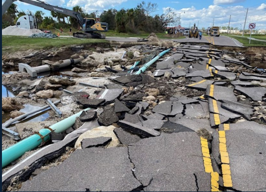
Road reconstruction of Price, Hillsborough and Chancellor Boulevards and more location
